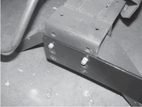
Figure 3-Left Side Plate installation
